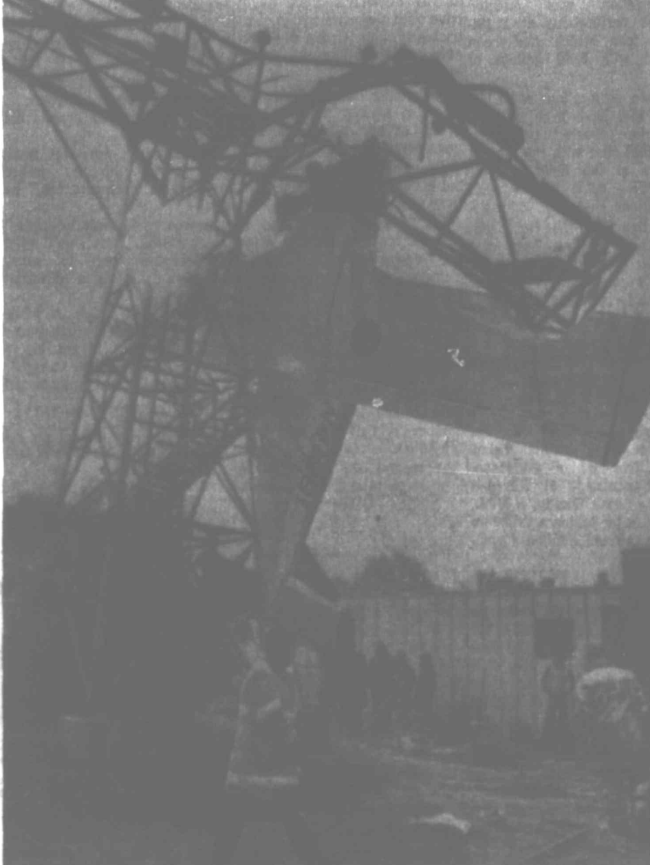
ONE-POINT LANDING—A light airplane hangs from a landing light approach tower, where it crashed while making an approach at Capital City Airport near Harrisburg, Pa., Sunday. The student pilot, alone in the plane, suffered only minor injuries. (AP Wirephoto.)
