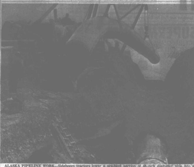
ALASKA PIPELINE WORK—Sideboom tractors lower a pre-bent section of 48-inch diameter pipe into a ditch adjacent to the Little Tonsina River north of Valdez as work goes on on the Trans Alaska pipeline. The pipeline is bent to conform to the contour of the ditch.
