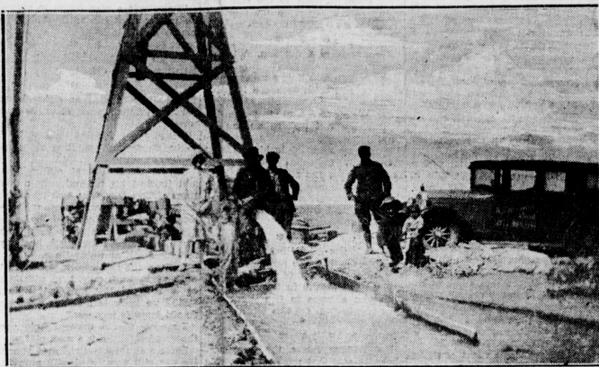
This new irrigation well, located on the old Steele Ranch, five miles south of Muleshoe, delivers 1,300 gallons of water per minute, according to tests made by the Dempster Pump Company. The land, now owned by Mr. Otto Stalley, of Austin, Texas, will be put on the market in forty-acre tracts within a few weeks. This well was drilled by H. J. McCarty & Son of Sudan, Texas, who, it is understood, will drill several others on this six-thousand-acre tract during the coming summer.
