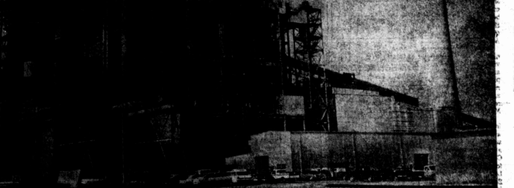
The 575,000 kilowatt Unit #1 at the new lignite coal-fired Monticello generating station is now in operation. Right behind it and still under construction is Unit #2, which will have the same capacity.
