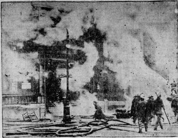
Ten persons were burned to death and others badly injured in a fire that destroyed a movie studio in New York. This picture of the conflagration was sent by telephoto.
