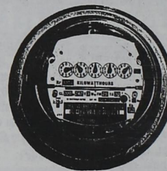
Conservation efforts are reflected in your electric meter, which measures energy use.
