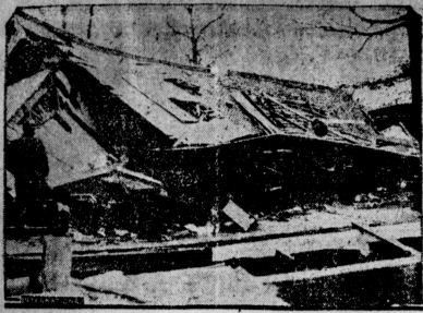
The ruins of the frame school building at Maunie, Ill., after the tornado which swept the Middle West. Two children, Dorothy Hambley, fourteen, and Berale Tucker, eleven, were killed in its collapse.
