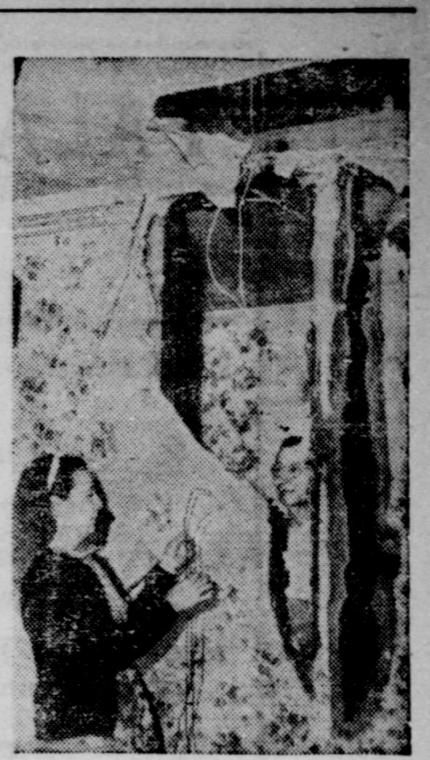
BOLT FROM SKY . . . Joseph Fey peers through aperture left in George Summacher home, South Gate, Calif., by bolt of lightning that traveled down TV antenna. California recently received rain, storm, snow, hail, sleet, thunder and sunshine.
