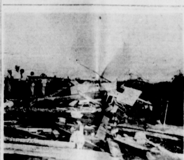
This is all that remains of the Rev. E. Peppy Blount's home. The twister that struck about 5 p. m. Tuesday leveled the building. Note Pup that stood guard over the demolished residence.
