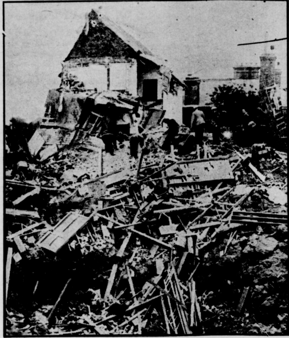
German planes bombed this house in a south coast English town, trapping a number of people in the wreckage. Note crater in foreground where heavy bomb exploded.
