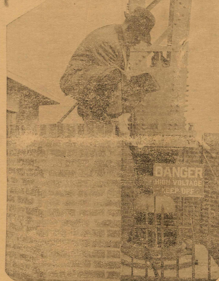
At the top left, Joseph A. Chambers, technical supervisor of radio station WLW, is seen drawing an arc, the flame in the photograph, from a strut with a lead pencil giving a rendition of the radio program audible for a distance of thirty feet. At the bottom, Chambers is drawing an arc with a pair of pliers from the iron gate protecting the base of the great WLW tower. The music was distinctly audible to persons 15 feet distant. At the top right is shown the device for carrying off lightning that may strike the tower. When the electricity jumps across the safety gap, the lightning is carried harmlessly to the ground. The power supplied the tower is so great that the arc would be continuous when once formed and drain all the power into the ground, but for the electric eye seen in the photograph behind the arc. For the photograph, the electric eye was disconnected temporarily permitting the arc to continue long enough to be photographed.
