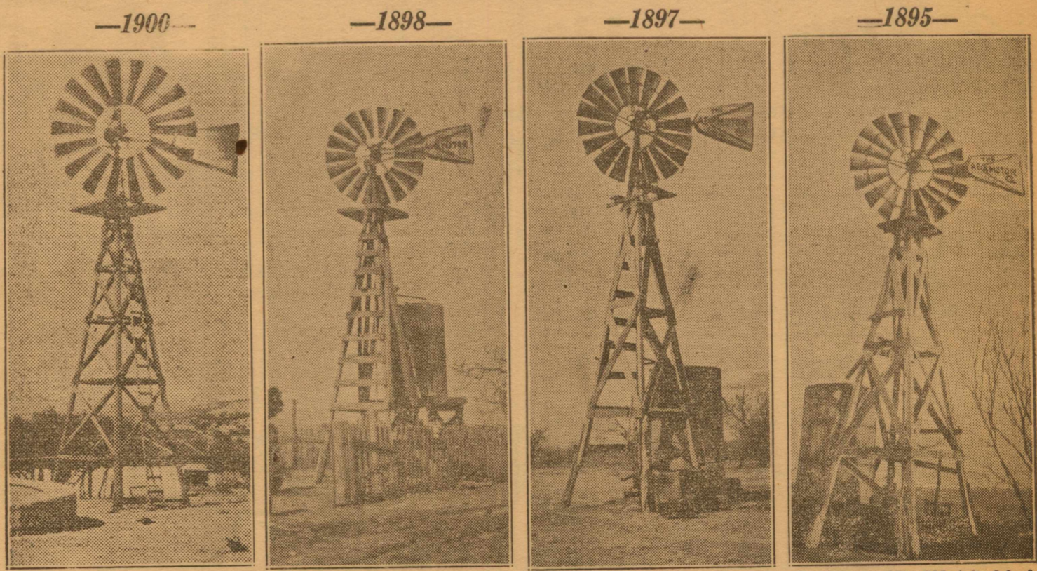
16-foot Aermotor on Word Ranch, Sutton County. Has seen continuous service since 1900. Now has self-oiling motor; original wheel and other parts.
