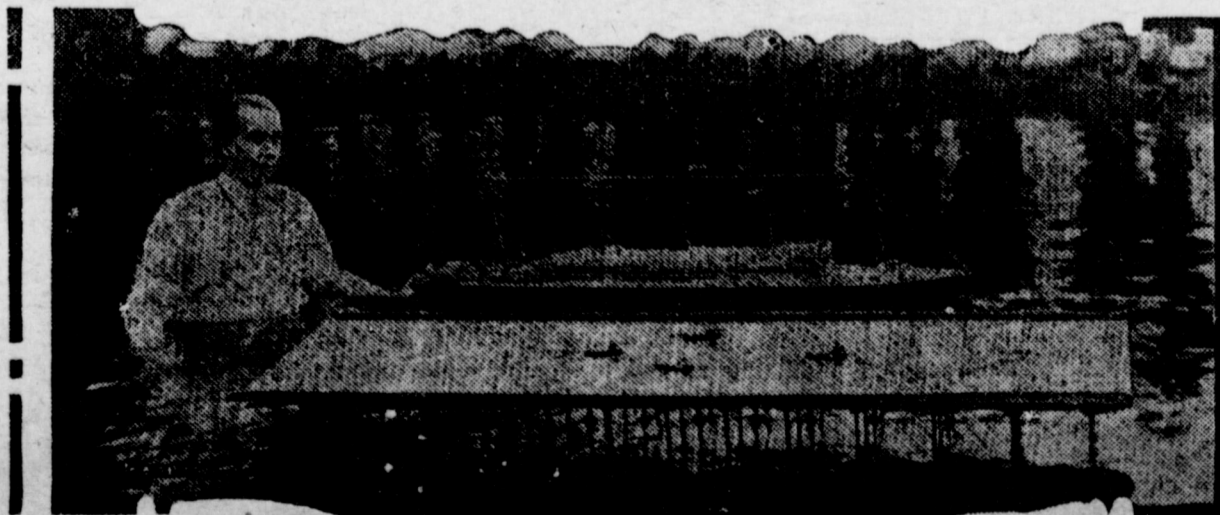
Above is pictured E. R. Armstrong, chief engineer of the Dupont company, with the elaborate model of his proposed seadrome, which he believes would solve the problem of transatlantic aerial travel. The drydock would serve as a midocean harbor for ships and dirigibles which could land on the dock. In the model he uses a replica of the S. S. Majestic, showing the relative sizes of the dock and the ship.
