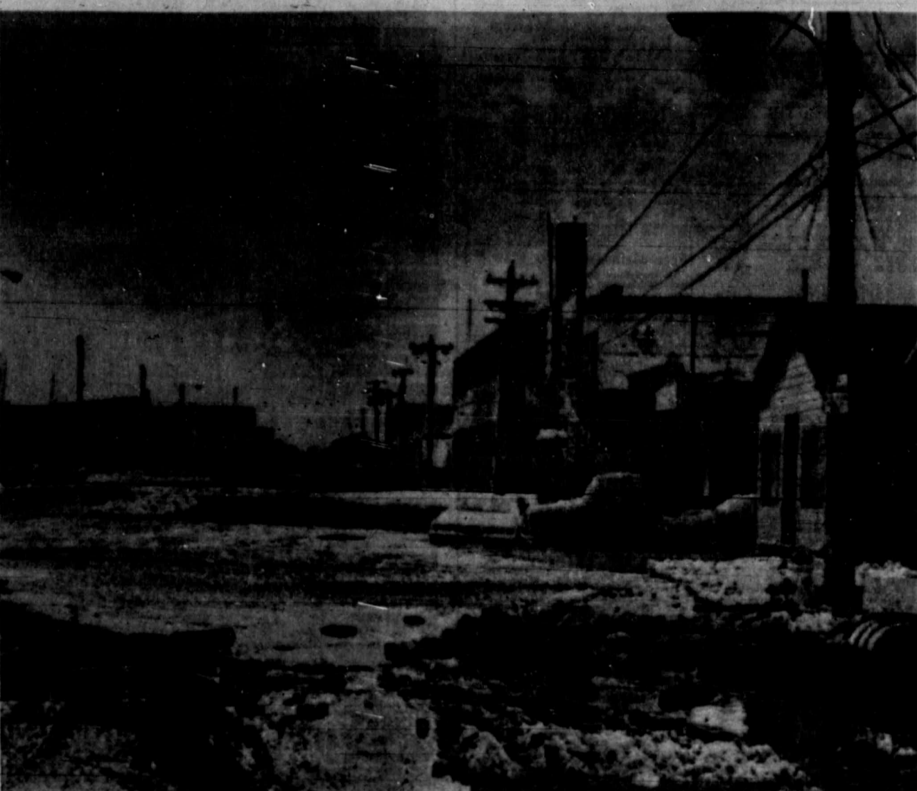
CLEAN-UP TIME — Front Street, the main thoroughfare in Nome, Alaska, is dotted by deep ponds and debris following a winter storm which at one time covered the town's business district with five feet of water. Alaska's Gov. William A. Egan has declared Nome and surrounding villages on the Bering Sea a disaster area and has asked President Ford for federal help. (AP Wirephoto.)
