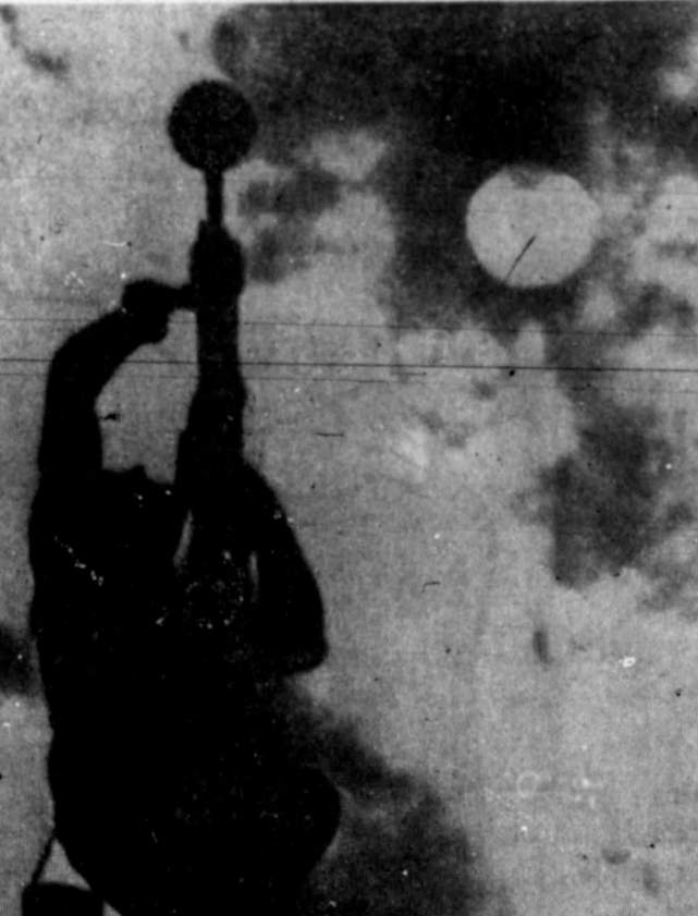
HIGH MAN ON POLE — Gerald Ogg of Columbus, Ga., is a professional painter of flagpoles who shuns conventional equipment. Ogg uses a harness with knots that will slide up the pole but not down. It holds him in place while he is working. (AP Wirephoto.)
