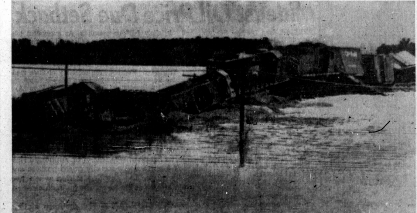
DERAILED BY FLOODWATERS — Floodwaters from heavy rainstorms washed out a track embankment along Hickory Creek near Belton, causing this freight train to derail. No one was injured in the mishap, but it will be several days before traffic can be resumed. (AP Wirephoto.)
