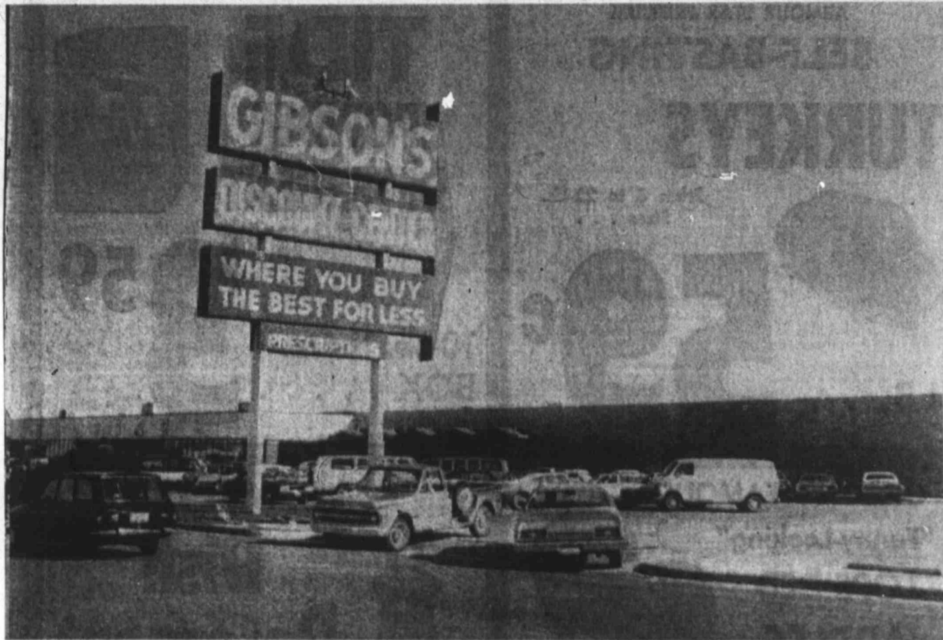
GIBSON'S COMPLETES EXPANSION—The area shown to the right of the sign recently was completed as a major expansion to Gibson's Discount Center. Ribbon-cutting ceremonies at 10 a.m. Wednesday will formally open the store's new area.
