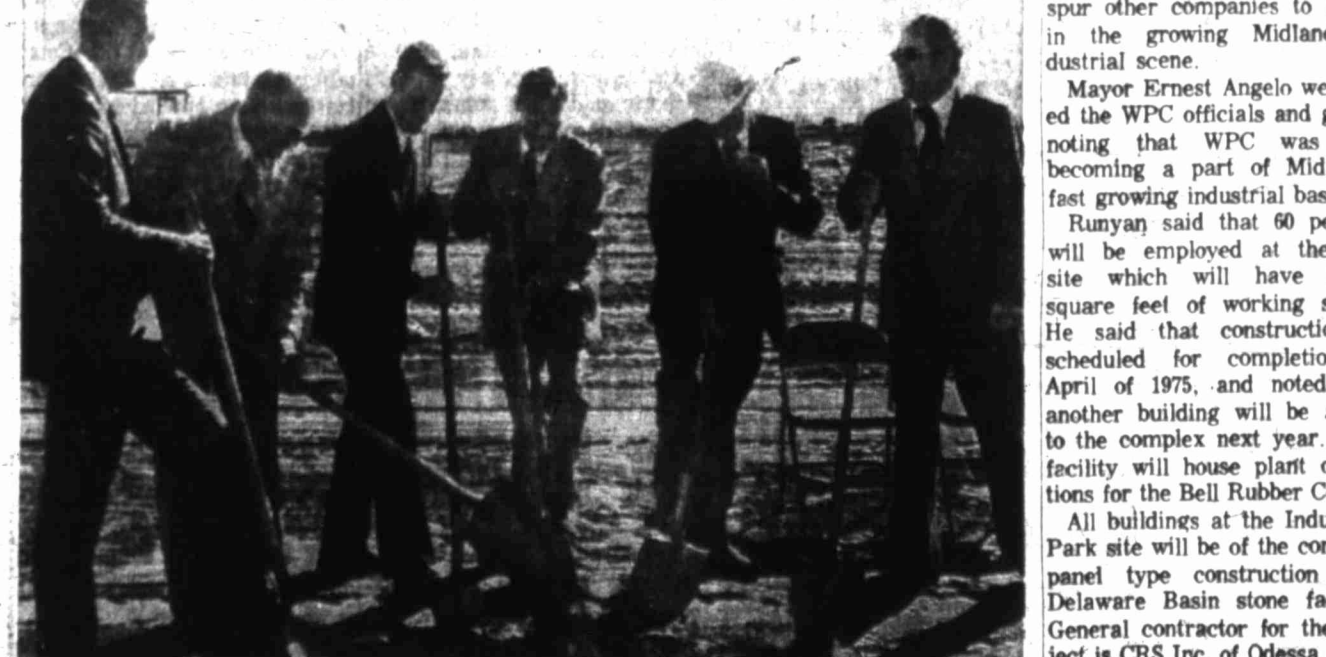
WPC GROUNDBREAKING — Tossing over the first spade-fuls of soil to symbolize the start of construction for Midland's newest oilfield service complex at Industrial Park, Western Pollution Control Inc., are, from left, E. E. Runyan, WPC president; K. M. Jastrow, president Midland Chamber of Commerce; Mayor Ernest Angelo; Win Brown, county commissioner; Charlie Welch, county commissioner, and Martin Allday, president Midland Industrial Park Development Corp. Completion of the three-building complex is scheduled for April of 1975.
