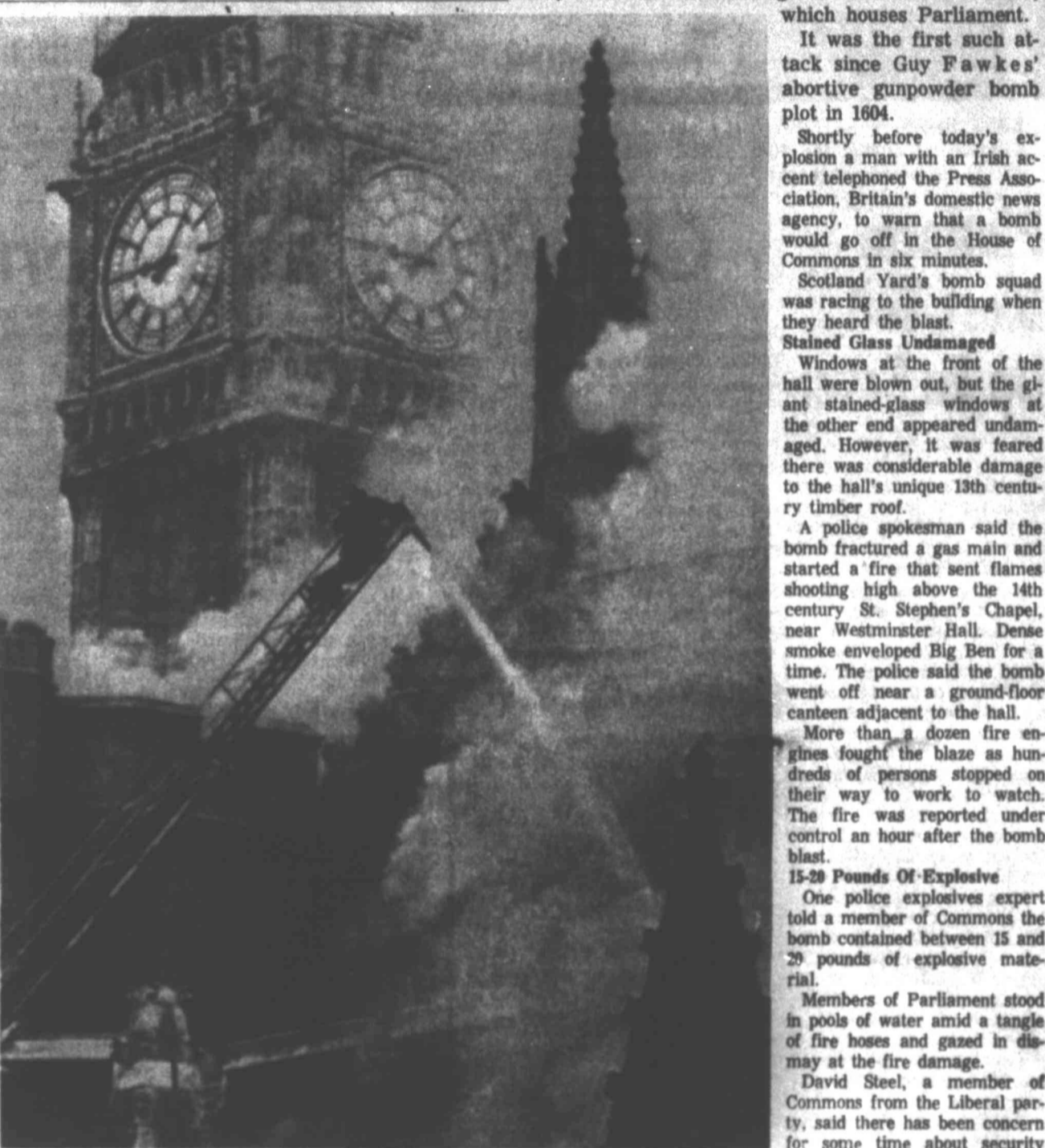
LONDON SCENE—Overlooked by Big Ben, the famous clock that dominates the tower of the British House of Commons, a fireman directs his hose onto the burning St. Stephen's Chapel after an explosion fired the building. At least 11 persons were injured by the blast and the blaze that followed. (AP Wirephoto.)
