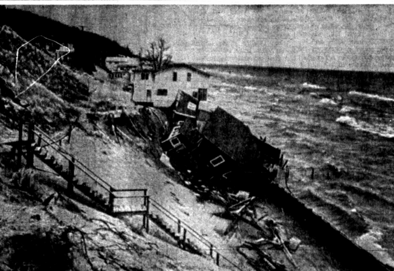
SMASHED BY WAVES — A summer cottage was smashed by high waves and swept into Lake Michigan in Grand Haven, Mich. Residents of the area say this is the fourth time in three years a cottage has been smashed by high water. (AP Wirephoto.)
