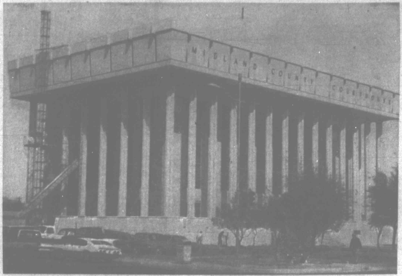
Midland County Courthouse renovation project continues
