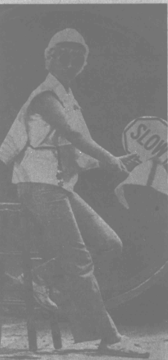
SITTING DOWN ON THE JOB — Women all over the country seem to be demanding their equal rights and Mrs. Olga Hamilton of Trinidad, Tex., seems to be getting hers and then some. Mrs. Hamilton is working at her new job, flagperson, for a construction company in Dallas and she has found a way to beat the old tired feet routine that so many flagpersons find. (AP Wirephoto.)
