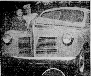
STRONGER "EYE APPEAL" is evident in the front-end design of the 1940 Plymouth at left. The photo shows how the fender "cat-walk" curves inward and up to form sides of bigger hood. Hood top now sweeps forward without a break to the new chrome-decorated grille, featuring larger louvre sections at the base where air-pressure is heaviest. "Sealed Beam" headlamps, that give 50-65% brighter road light, are streaming into the fenders and separate parking lights are built into the headlamp mountings.
