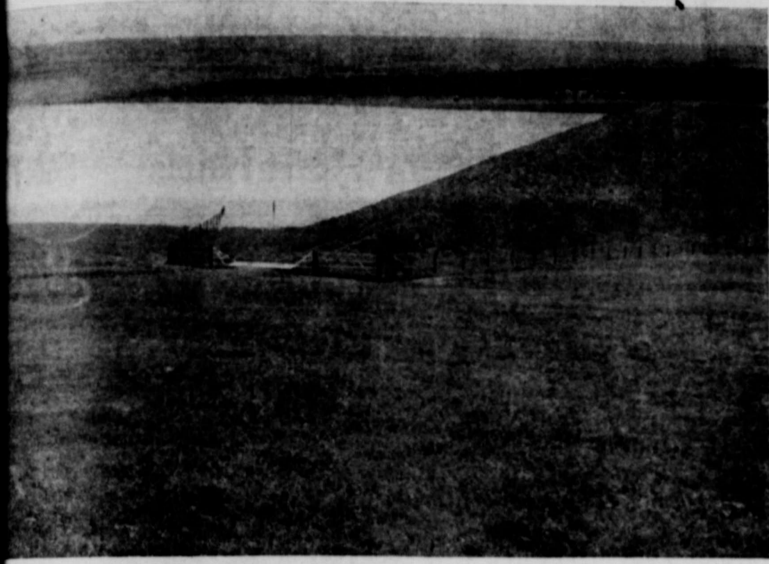
POLLUTION CONTROL —Structures such as the one in the top photo have greatly curtailed wash-outs as shown in the photo at left, and have been instrumental in halting flooding in the Bosque Valley. The upper structure is one of 26 constructed in the Upper Bosque River Watershed. The photo at left was made several years ago at Clairette after a damaging flood had taken its toll in the watershed. The flood control structures were credited only this week with preventing thousands of dollars in damages after heavy rainfall along the Bosque watershed.
