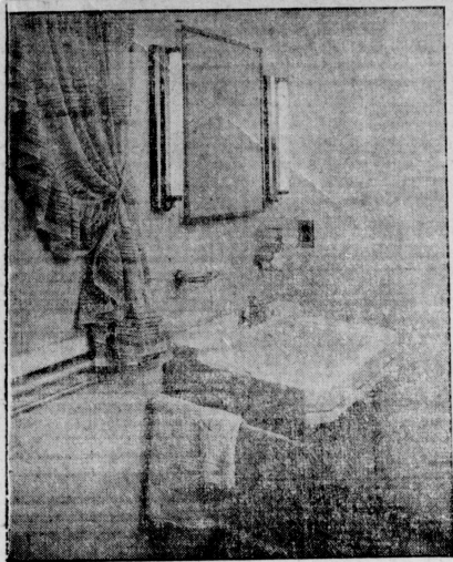
The tubular bulbs used of this mirror are the new fluorescent lamps, which closely simulate natural daylight.
