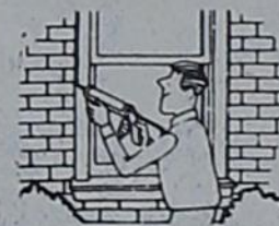
Caulk around doors and windows
