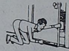
Weatherstrip all outside doors
