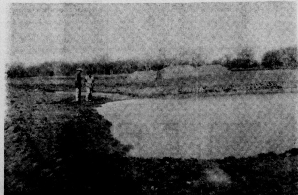
STORAGE—Water from the 700-gallon per minute well is ditched to this storage tank, which in turn will be pumped to various portions of the field.
