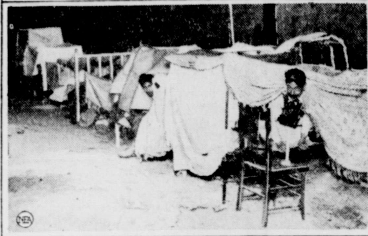
The earthquake that struck the thriving mountain city of Oaxaca, Mexico, recently, destroyed hundreds of homes and made thousands of people homeless. These photos show how refugees are being cared for. They are made-shift lean-tos, constructed in the open, to provide a little shelter for homeless families; below, a dormitory in the open street where men use beds and curtains to protect themselves from the elements.
