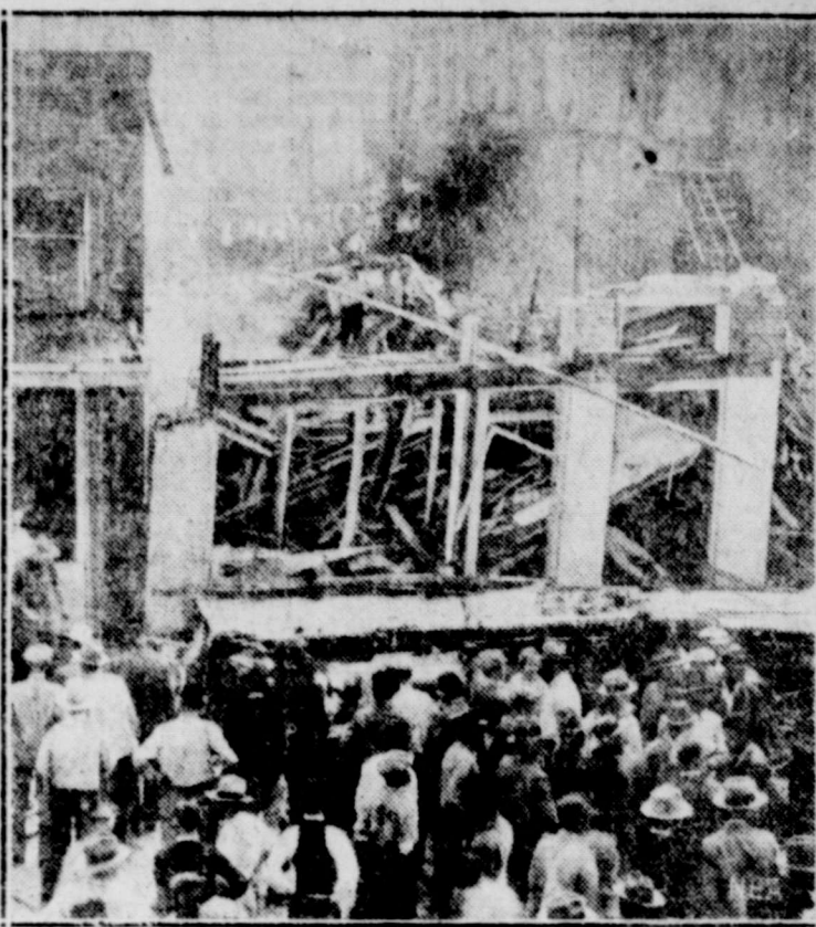
One man was killed and six more were badly hurt when a sudden explosion demolished the Macomber building in Palestine, Texas, causing damage estimated at $100,000. This picture shows how the wreckage looked. Cause of the explosion has not been determined.
