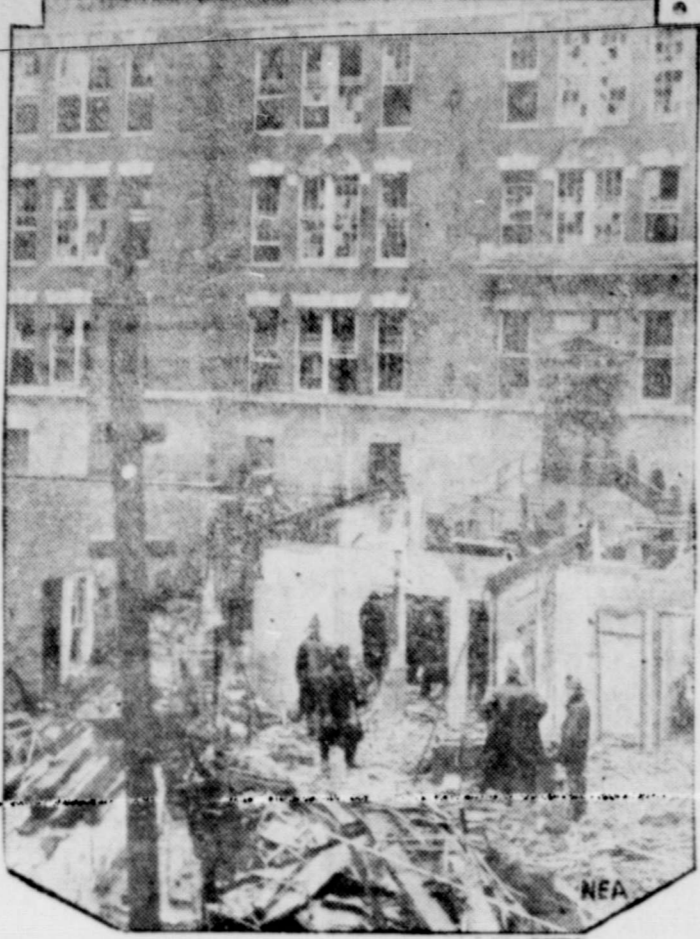
Like a scene on a war-torn battle front is the one pictured above after an explosion of accumulated gas had wrecked a frame in Bocklyn, N. Y., and wrecked the school building shown in the background, injuring more than 30 pupils. Many of whom were taken to hospitals. Here you see how roofs and walls of the building and the windows of the school were shattered by the terrific blast. Two thousand pupils were attending classes when the explosion occurred.
