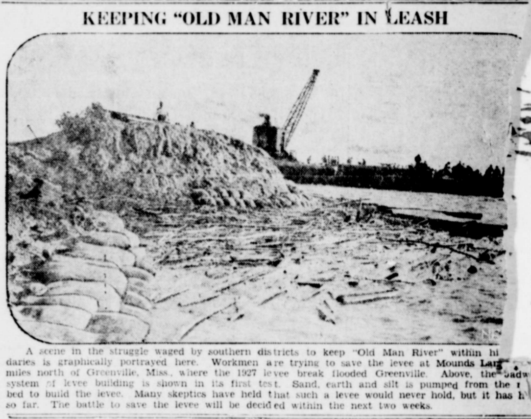
A scene in the struggle waged by southern districts to keep "Old Man River" within his daries is graphically portrayed here. Workmen are trying to save the levee at Mounds Lake, a miles north of Greenville, Miss., where the 1927 levee break flooded Greenville. Above, the sledge system of levee building is shown in its first test. Sand, earth and silt is pumped from the bed to build the levee. Many skeptics have held that such a levee would never hold, but it has held so far. The battle to save the levee will be decided within the next two weeks.
