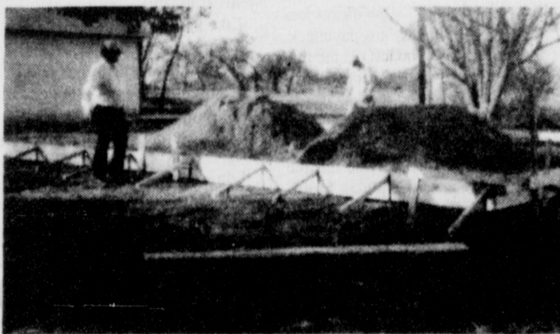
CONSTRUCTION ON COVERED PAVILION BEGAN
