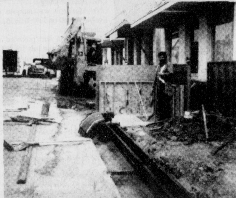
SIDEWALK PROJECT CONSTRUCTION UNDERWAY IN DOWNTOWN CROSS PLAINS
