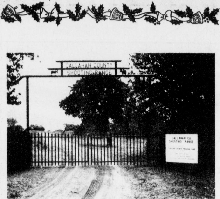
SHOOTING RANGE ENTRANCE —Pictured is the entrance to the Callahan County Shooting Range which is nearing completion. The range
