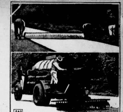
SCOTT, Miss., . . . The first "Cotton Highway", a 14-mile experiment in road construction is rapidly nearing completion here. The upper picture shows the cotton fabric membrane being rolled out on the highway on a base of mixed clay and gravel. Lower picture shows coat of tar over cotton, this covered with two applications of asphalt mixed with screen gravel.
