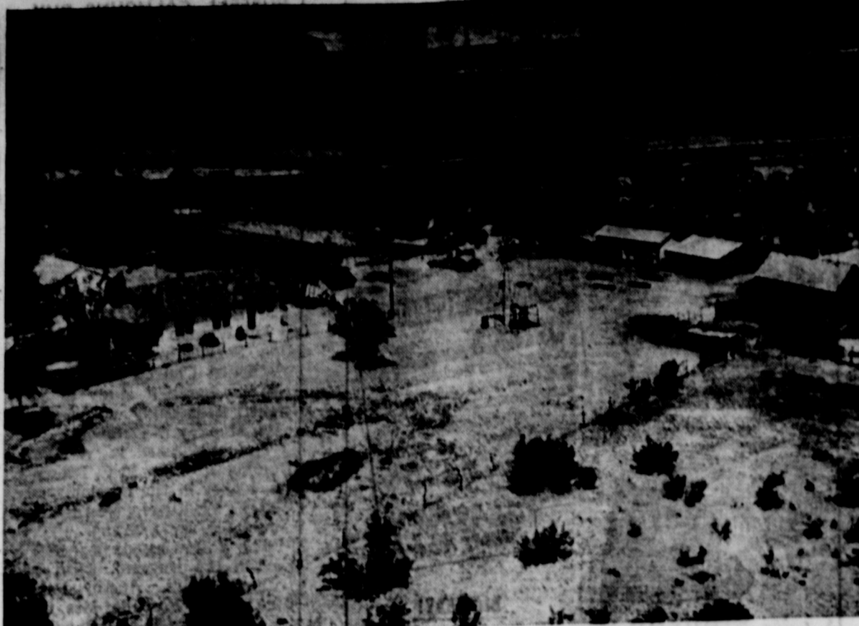
RECOGNIZE THIS PLACE? The aerial shot of the home above is another in a series of country homes which have
