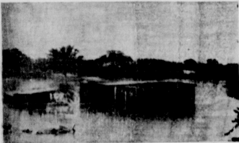
Home of Charlie Baugh inside city under three feet of water
