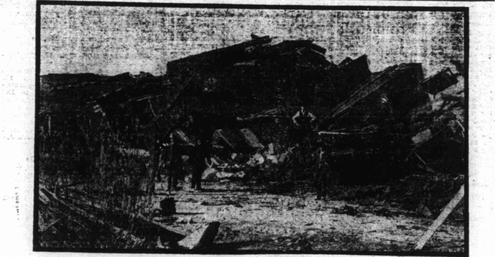
Here is a freak wreck, even for Texas, where freight train wrecks are no more unusual than in other states. The picture shows seventy-five feet of space, in which were piled twenty-one freight cars, which were wrecked on the Fort Worth & Denver Railroad between Amarillo and Channing a few weeks ago. Two men and seventy-six horses were killed in the wreck.
