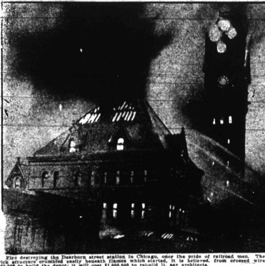
Fire destroying the Dearborn street station in Chicago, once the pride of railroad men. The wood and brick structure crumbled easily beneath the flames, it is believed, from crossed wires. It cost $200,000 to build the depot; it will cost $1,000,000 to rebuild it, say architects.
