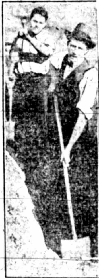
Not content with digging up funds for the new Fifteenth Street Christian Church, Washington, D. C., the pastor, Rev. J. N. Jarrett and his congregation intend to complete the digging for the foundation before turning the work over to the contractor. Rev. Jarrett is shown wielding a shovel.
