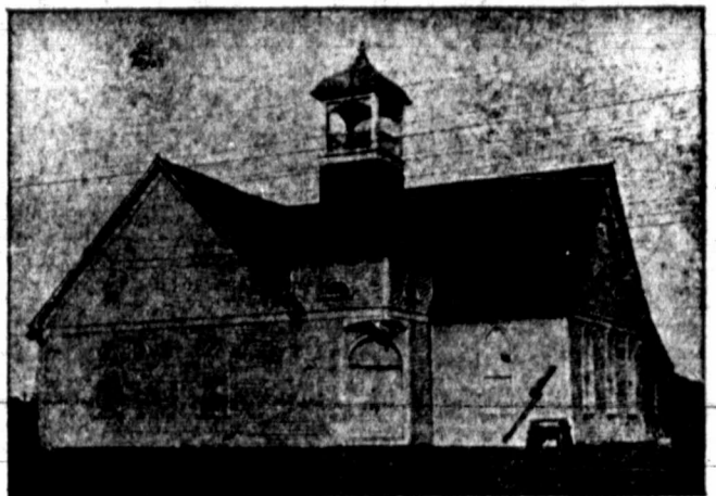
Building inadequate for present needs.
