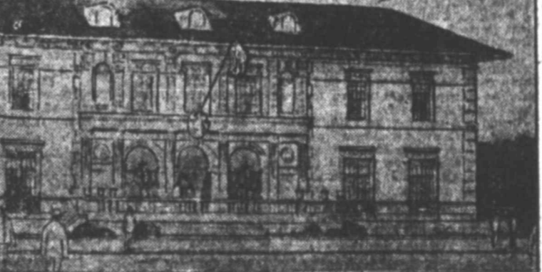
United States Government Building being erected at Rio de Janeiro in commemoration of America's part in the Brazilian Centennial Exposition. A temporary structure will adjoin this building on the rear, the whole to be used to house the Federal exhibit during the exposition, September 7, 1922, to March 31, 1923, after which the permanent building shown here will be used as the United States Embassy.
