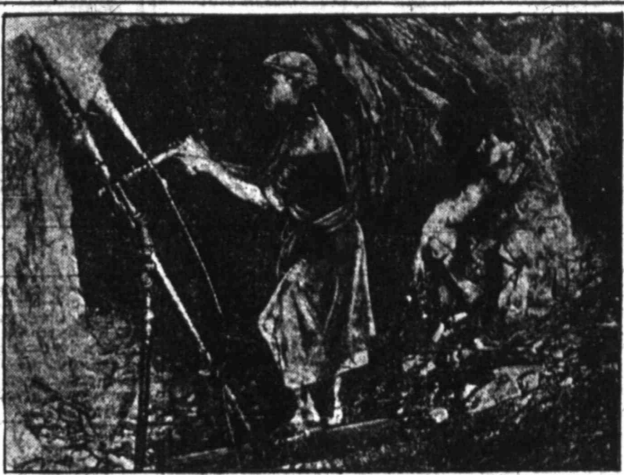
Operating an electric drill in a South African gold mine
