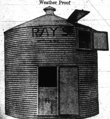
These bins are made of the best galvanized sheets, they are equipped with two doors in side and manhole in roof, all weather proof, also ventilator in roof through which heated air passes to outside,
