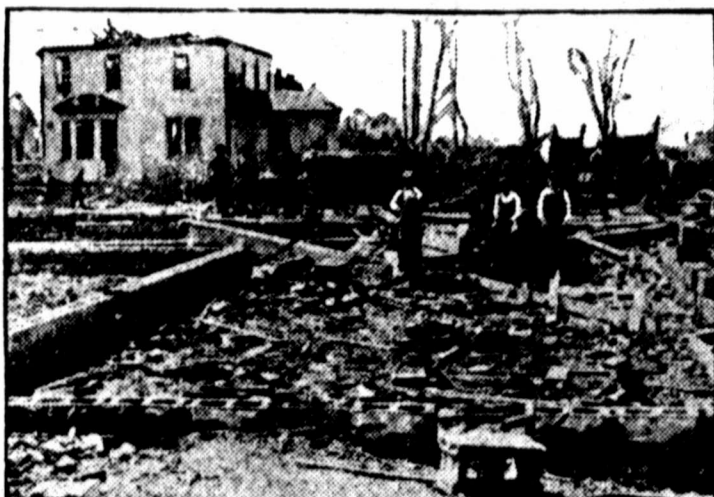
The Illinois tornado tore the Irvington school from its foundations and literally scattered it all over town. Not even a whole desk could be found. Had the tornado occurred in the daytime, many of the students undoubtedly would have been killed.
