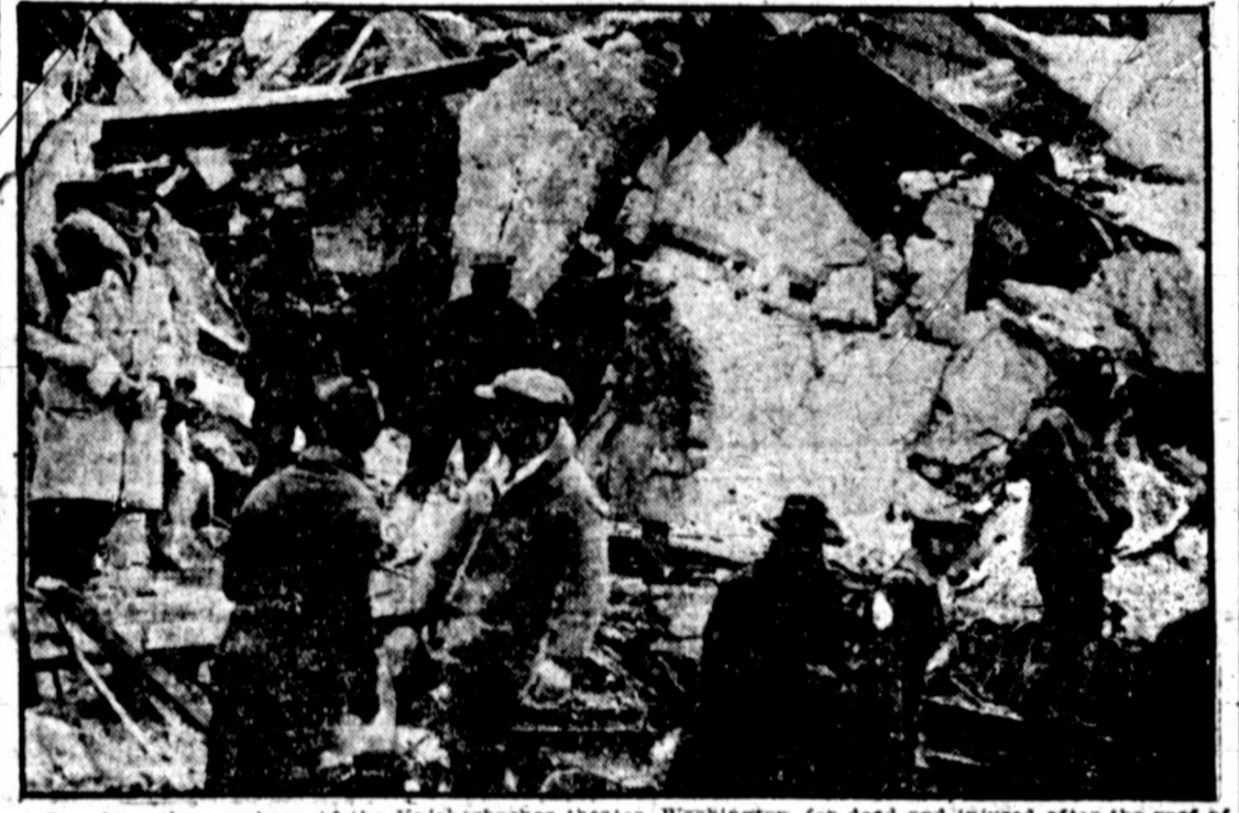
Searching the wreckage of the Knickerbocker theater, Washington, for dead and injured after the roof of the fashionable motion picture house collapsed, killing and injuring more than 200. Firemen, soldiers and citizen volunteers are shown at work. Note the massive steel girders which supported the roof and the great blocks of concrete that fell when the girders gave way under the weight of snow. At the left one of the broken girders can be seen.
