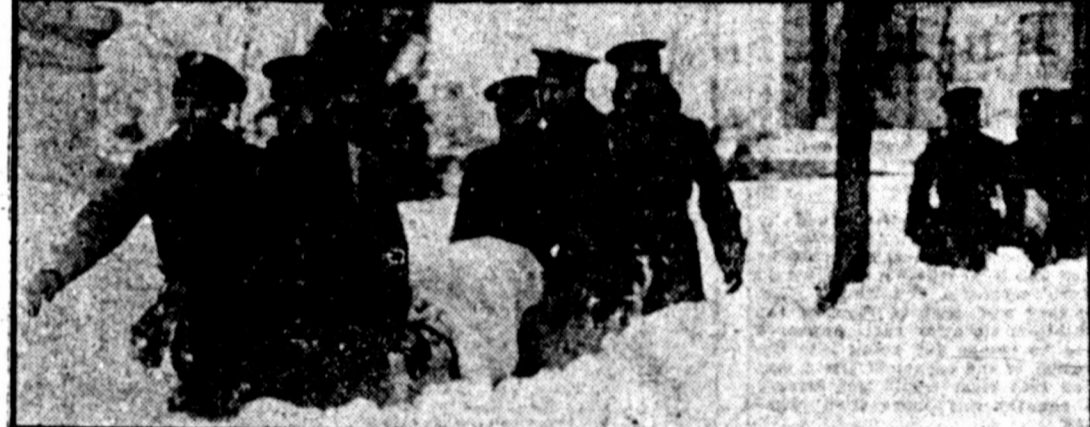
Groups of soldiers removing two of the victims from the Knickerbocker theater, Washington, where 20 were killed and more than 200 hurt when the roof of the snow which is thought to have been responsible for the collapse of the theater roof.
