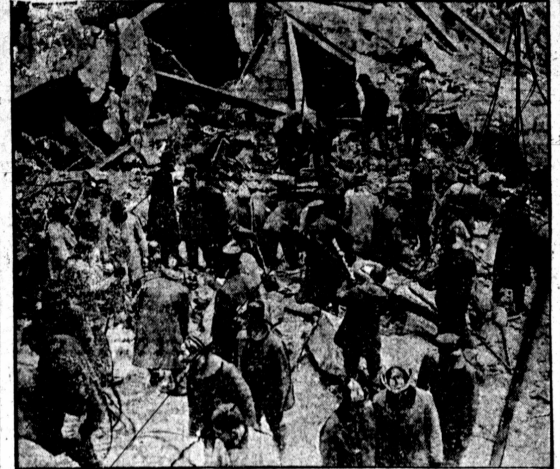
This close-up view of the ruins of the Knickerbocker theater, Washington, D. C., gives a definite idea of the proportions of the wreckage. Soldiers, firemen and civilians are probing in the ruins to locate the dead and the injured. In the center group are two stretcher-bearers carrying a victim to one of the many ambulances awaiting outside.
