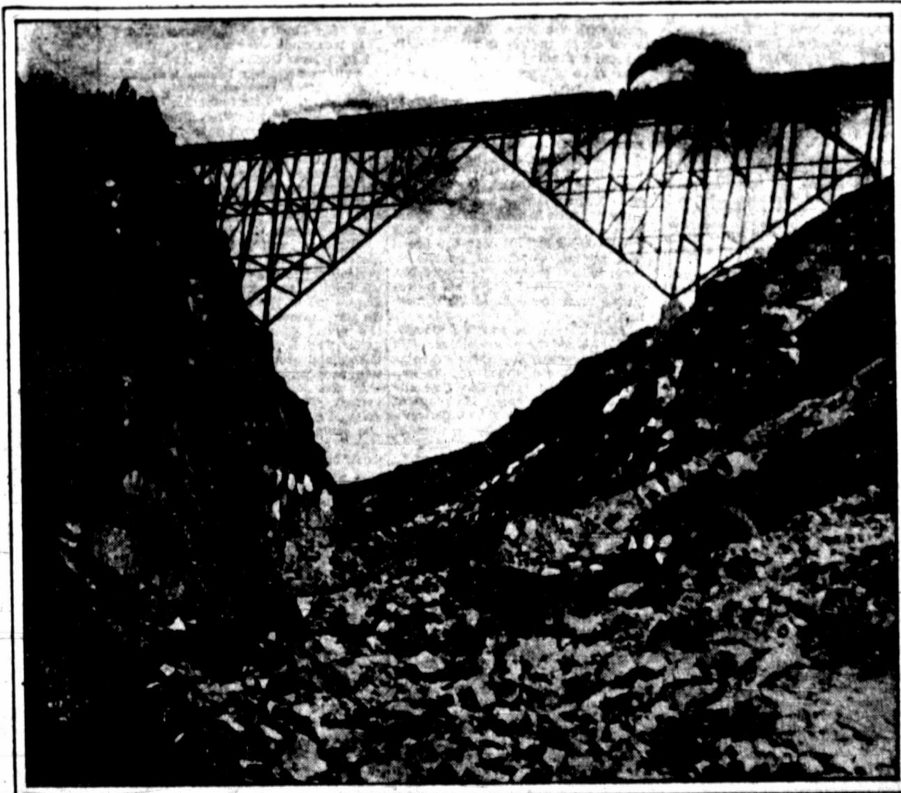
One of the gigantic chasms spanned by a web of steel along the right of way of the Alaskan railroad
