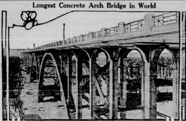
One mile in length with 12 piers 120 feet high, the new Mendota bridge at Minneapolis is the longest concrete arch structure in the world and cost \$2,000,000. It was dedicated to war heroes. There is a roadway of 43 feet width over which pass many thousand vehicles each day.
