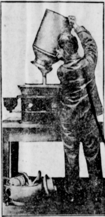
Each Dairy Farm Should Be Equipped With an Inexpensive and Serviceable Sterilizer Such as Is Shown.
