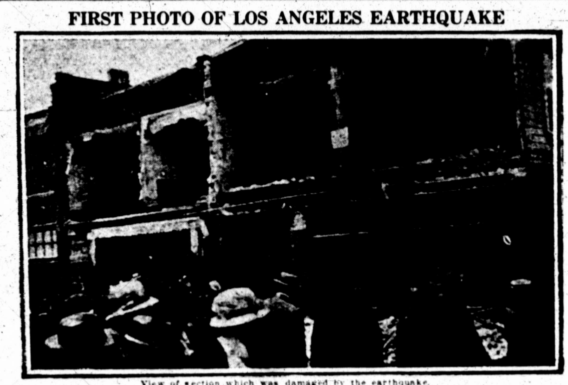
View of section which was damaged by the earthquake.
