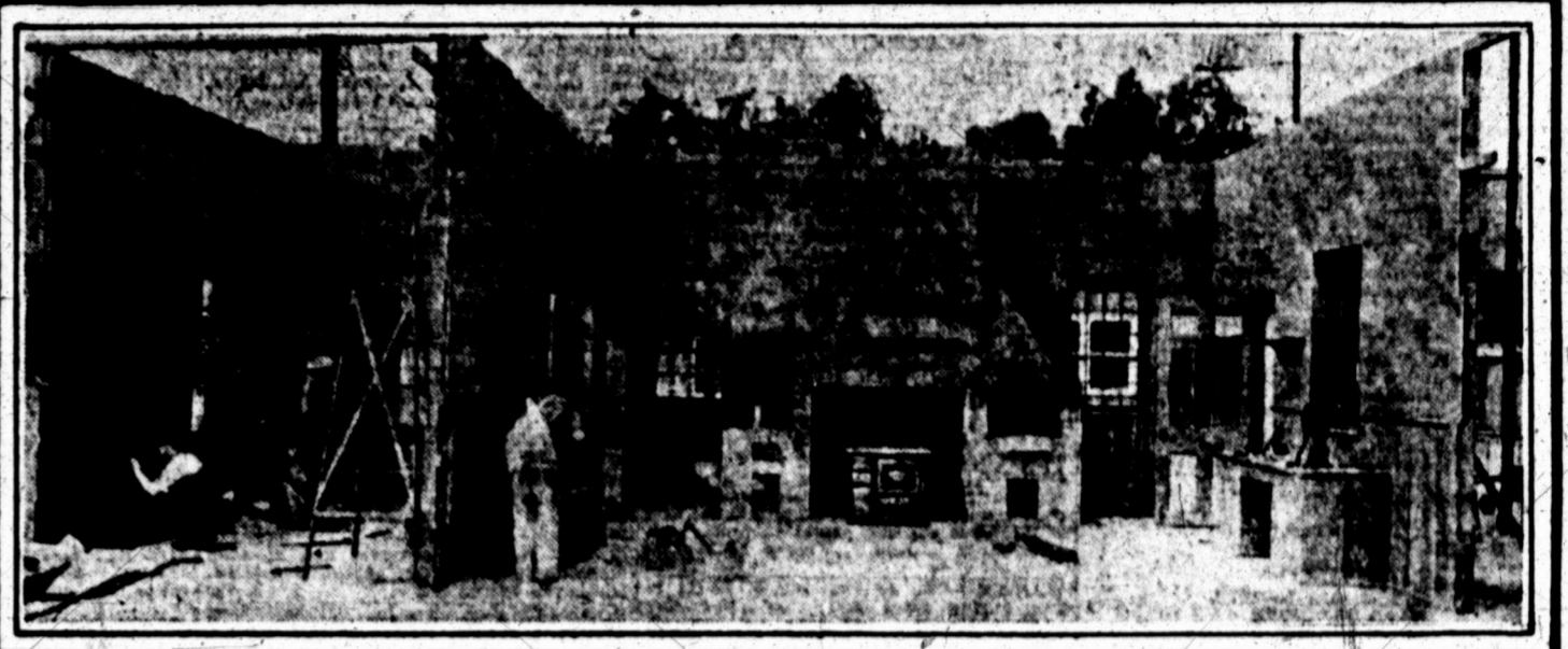
Set of Kitchen-in Mansion-During Construction
